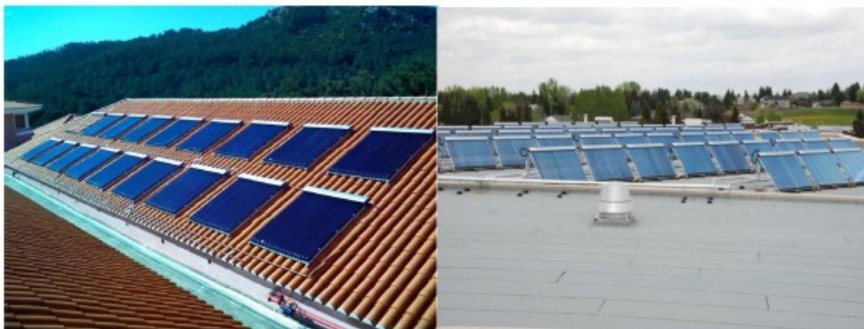
Spain: Alcomer swimming pool heating 70 m 2 2008
